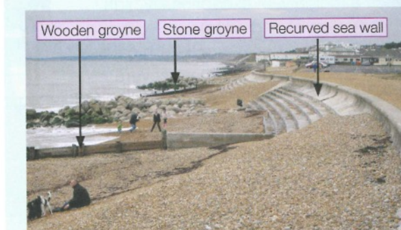
Figure 2 Milford-on-Sea. Coastal management has affected the coastline by trapping sediment.
