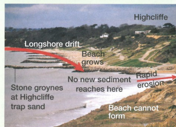
Figure 2 The stone groynes at Highcliffe have built up the beach, but have caused rapid erosion downdrift. This is called terminal groyne syndrome .
